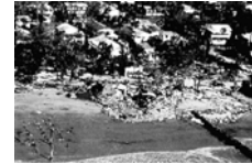
A section of shoreline after storm surge at Folly Beach, SC
