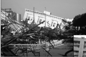
Loma Prieta, California, Earthquake October 17, 1989. San Francisco. Photo Credit: USGS
