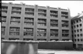
Latimer Hall, University of California at Berkeley after seismic retrofit.
