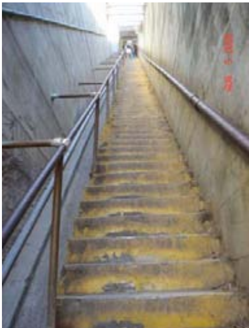
Photo 7: This stairway had 99 steep stairs to climb.
